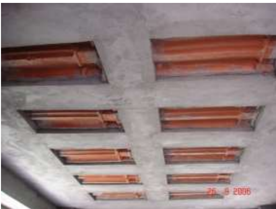
Figure 14: FILLER SLAB
