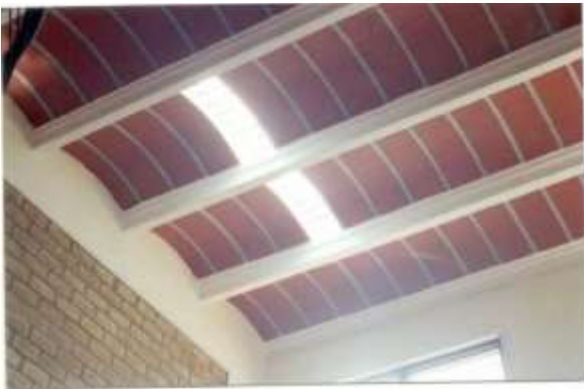
Figure 16: PRE-CAST ARCH PANEL SYSTEM
