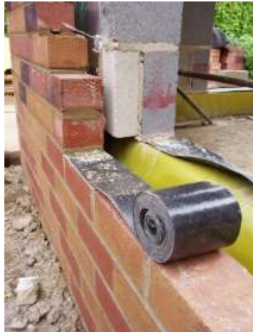
Figure 20: DAMP PROOF MEMBRANE
