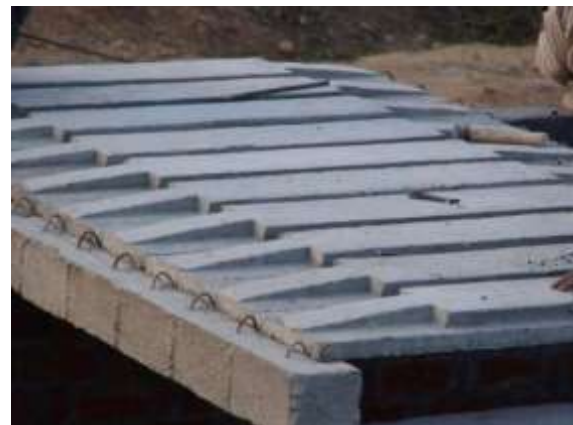
Figure 15: PRE-CAST RCC PLANK AND JOIST
